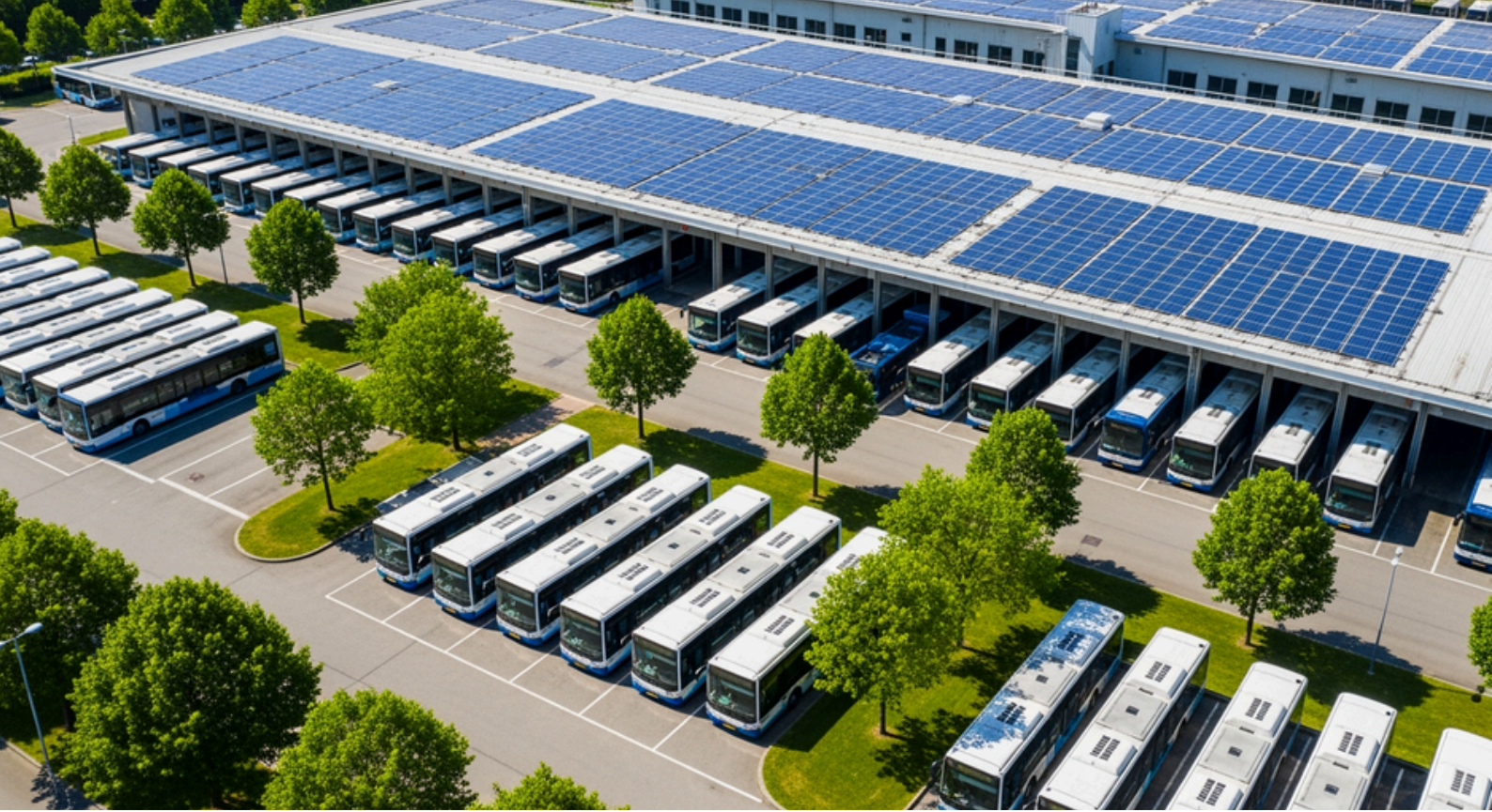
Fig. 1: E-bus depot with a photovoltaic system and battery storage.
